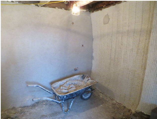
Second coat (left) being applied on top of first coat (right); HES image
