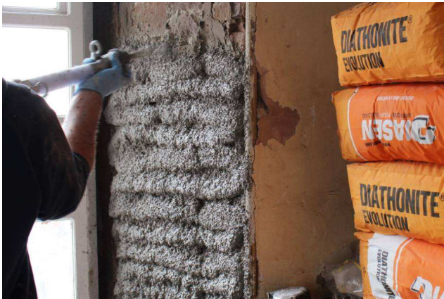
Spray application of insulated lime plaster © Ecological Building Systems
