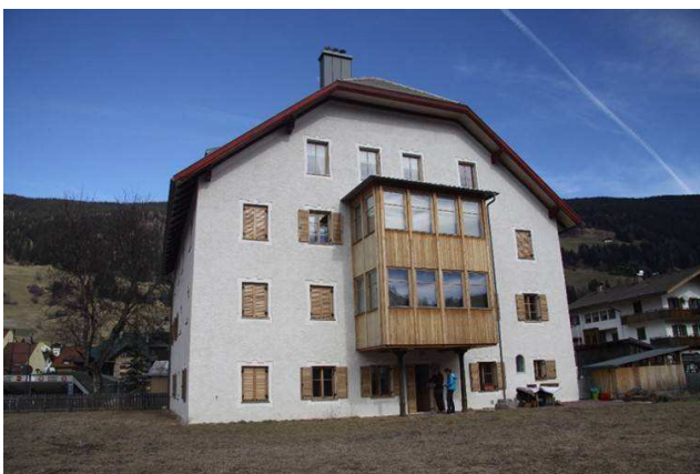
External view of the completed renovation
