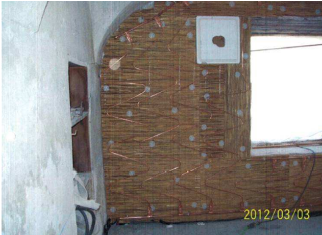
Construction phase - internal insulation + radiating wall heating
