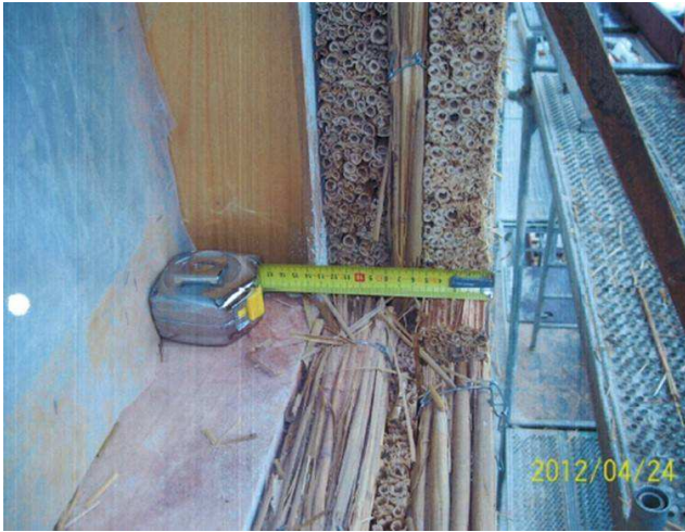
Construction phase - external insulation thickness
